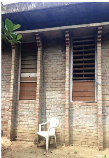
Fig. 7: Tradional Timber Louver window
