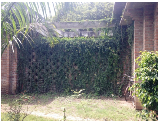
Fig. 10: Creepers used over Brick jaali for better climatic control
