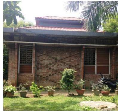
Fig. 11: Cross cross pattern of brick wall
