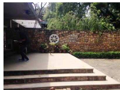
Fig. 12: Stone wall acting as Thermal insulator
