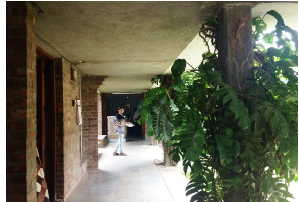
Fig. 4: Semi open corridors highlighted through brick piers
